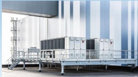
(Air Cooled Chillers)
